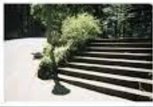
Portland: Access Barrier
